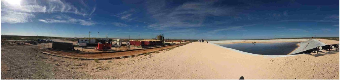
Figure 1. 6: PW treatment and pit storage facility in Southeast New Mexico.
